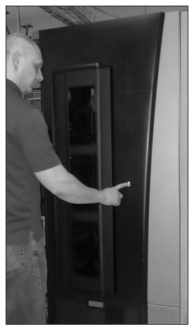
**Figure 234** Press the door release button to open the door.
